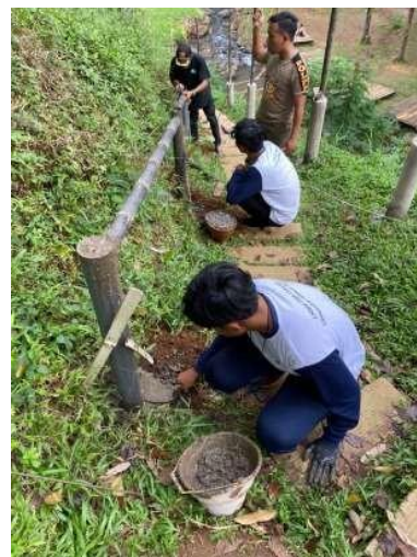
Picture 5. Installation of Staircase Handrails for Access to the Camping Ground.
